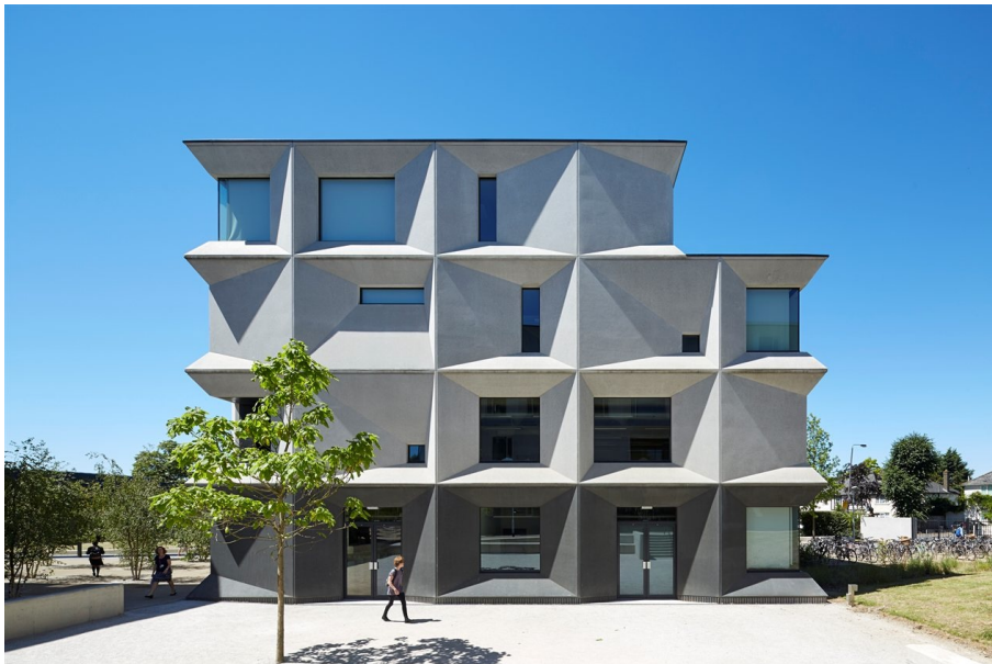
Burntwood School, Tooting winner of the 2015 RIBA Stirling Prize, the UK's leading architecture award (architects Allford Hall Monaghan Morris)
